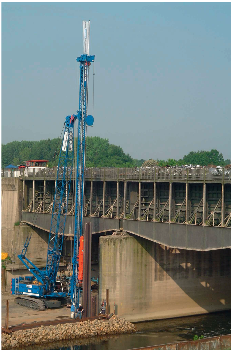
Hanging lead MH 35104 with diesel pile hammer D25-32 at the Dortmund-Ems channel in Germany
