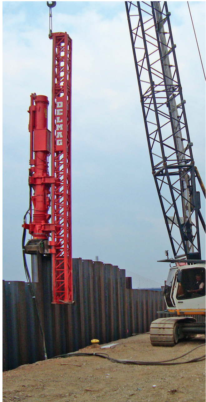
Diesel pile hammer D30-52 with swinging lead MS 32103
