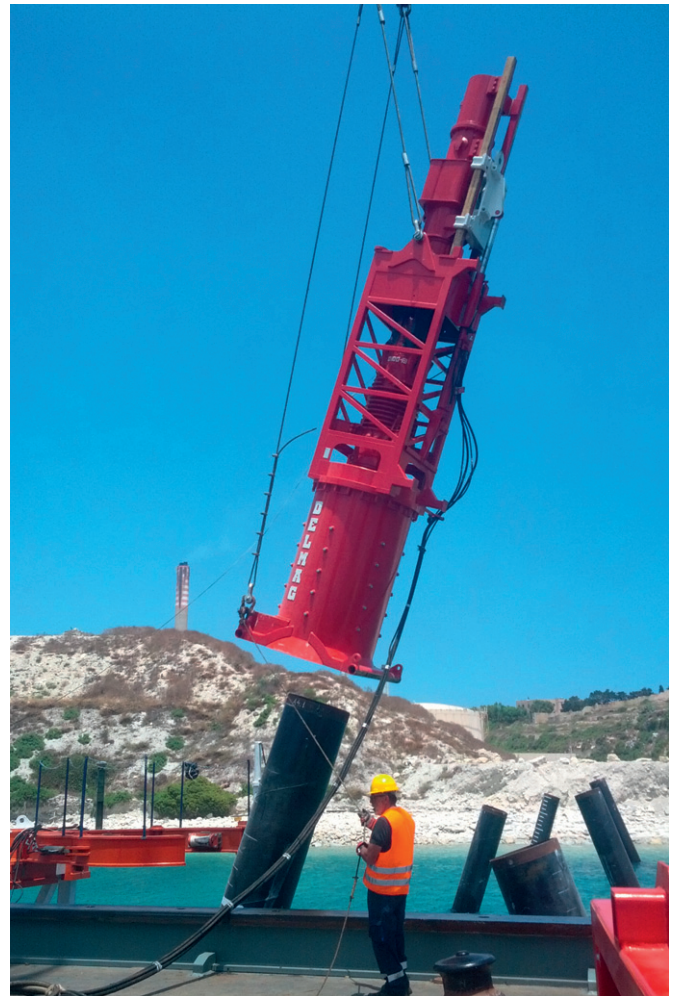
Diesel pile hammer D100-13 with rope suspended lead MAR 100-60
