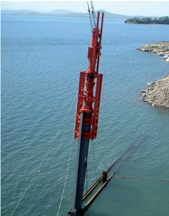
Rope suspended lead MAS 3000 with diesel pile hammer D25-32 in Russia
