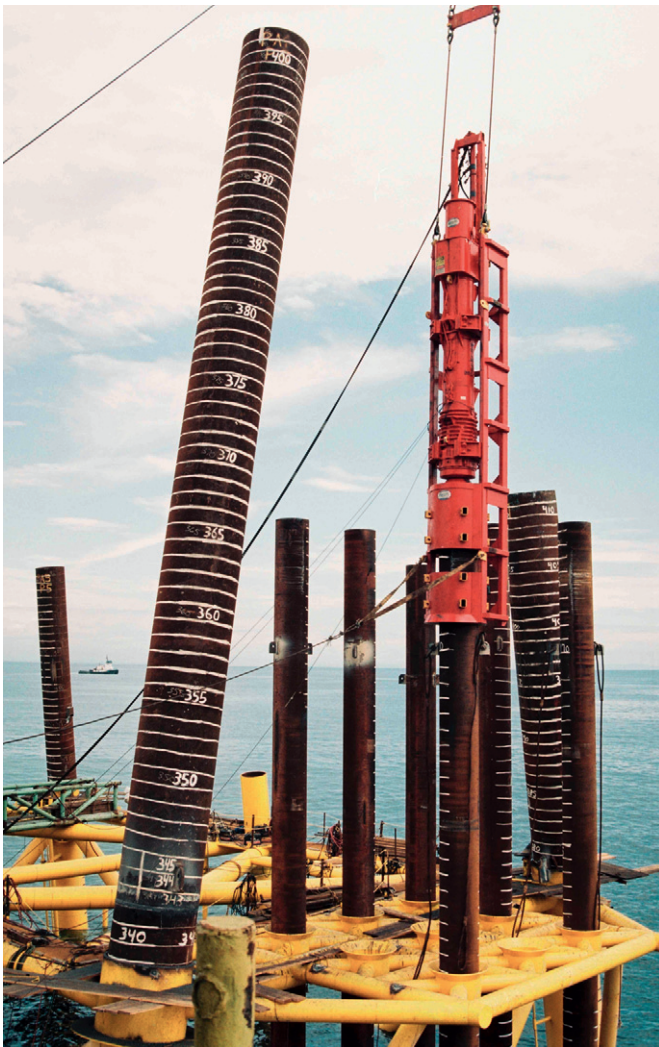
Diesel pile hammer D62-22 with rope suspended lead MBR 62-48
